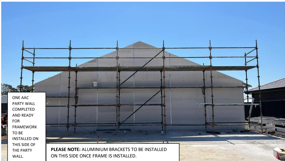
COUNTER-LEVERED SCAFFOLD USED TO COMPLETE THE WALL IN ONE SITE VISIT
